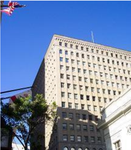
490 Post Street Exterior
